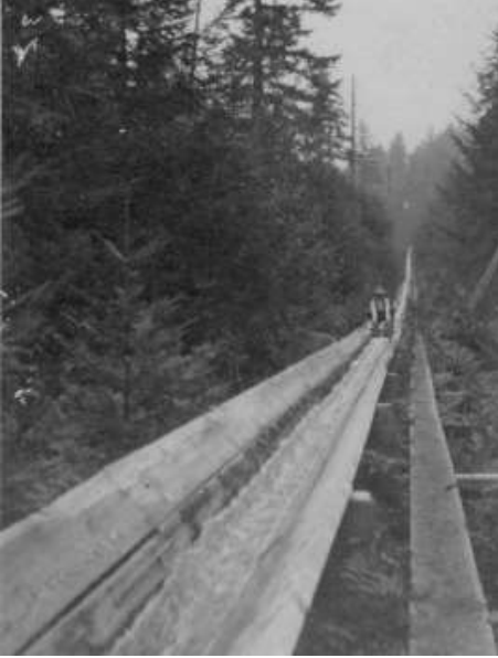
Flume that brought lumber from Prune Hill into Saginaw
